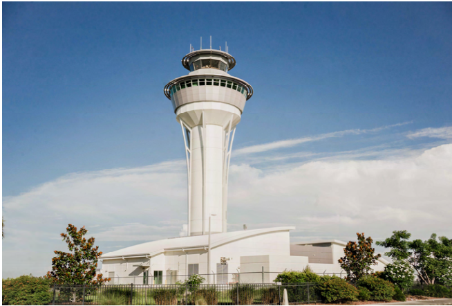
New Airport Traffic Control Tower Source: Lee County Airport Authority
