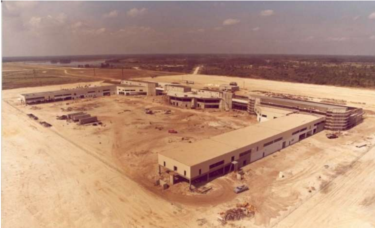
Original 1983 Terminal under construction Source: Lee County Port Authority
