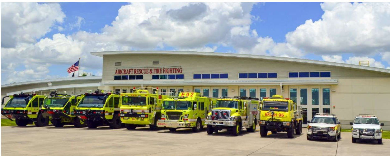
ARFF Station and part of the emergency response fleet Source: Lee County Airport Authority
