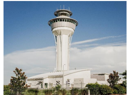
New Airport Traffic Control Tower
