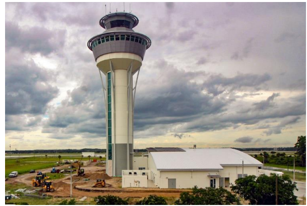
Future Airport Traffic Control Tower
