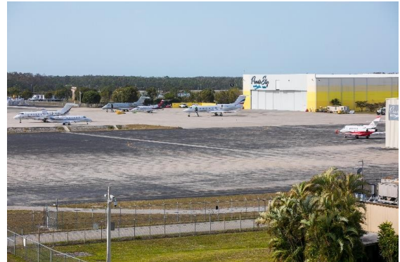
Private Sky Aviation Hangar and FBO/GA Apron
