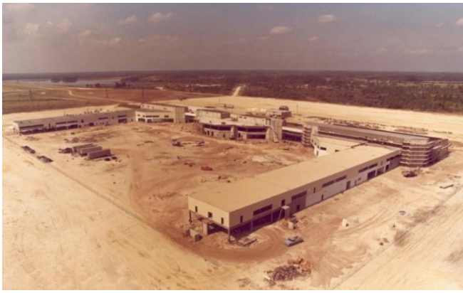
Original 1983 Terminal under construction
