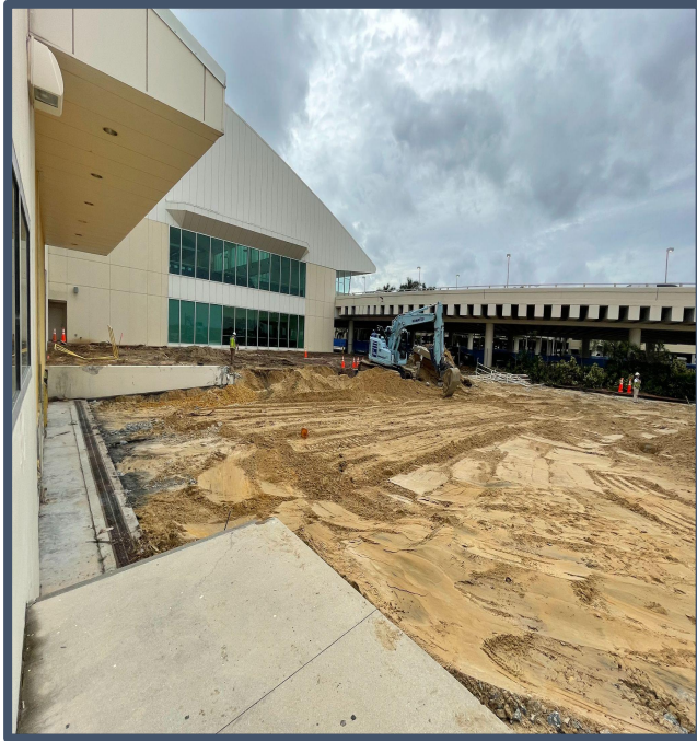
Apron Concrete Removal
